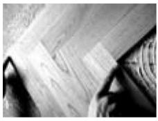
1. Once the sub floor has been deemed suitable for this installation, is flat and dust free, your floor can be set up for fitting, in the case of a herringbone and mitered herringbone, the installation needs to be started from the central axis, for straight lay typically the longitudinal side of the flooring should run across to the longitudinal side of the room this has the effect of making the room larger.
