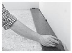
1. Cut the first row to size, centre and align the planking to the area
