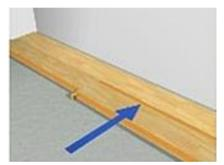
6. Use a hard striking block to close the long side joint, do not force the boards together move out the wedge and place it under the next board.
