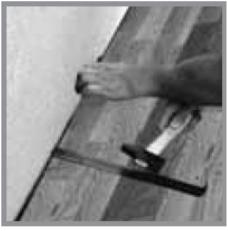
6. The strips for the final row will need cutting to width making sure that the expansion gap is allowed for. The use of a pull par or joint puller will be needed for this final row, wedges can be removed 24hrs after laying.
