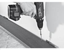
The planks in the first and last rows are fixed from the top with either nail or screw, the fixing is placed around 15mm from the edge of the plank
