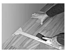
4. The positioning of wedges between the plank and the wall will allow an expansion gap all around the edge of the room, a minimum expansion of 10mm needs to be allowed, for larger rooms this needs to be increased, continue to lay your floor checking regularly for alignment and squaring if required.
