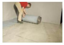
1. Roll out the underlay over the polythene moisture barrier in rows next to one another (the underlay strips must not overlap)
