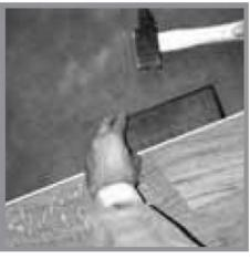
5. A tapping block will avoid any damage to the tongue while the strips are being fitted together
