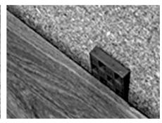
6. Fitting the final row will require the use of a pull bar or pulling iron this specialized tool makes up part of the solid wood / engineered fitting kit along with wedges and a tapping block. The wedges placed around the edge of the floor to maintain the expansion gap can be removed after 24hrs.
