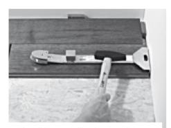
7. A pull bar or pulling iron can be used to help seat the end planks effectively
