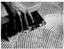
2. With a 6mm wood floor adhesive trowel the flooring adhesive is spread in a criss-cross pattern onto the sub floor as seen in the picture its advised to work on small areas at a time. Your wood floor adhesive will yield about 1m2 of coverage to 1000g of adhesive.
