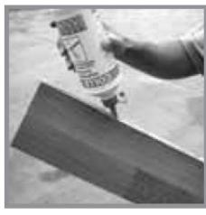
3. Apply glue to the upper edge of the tongue to the end or head joints as well as along the length of the first row.
