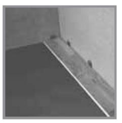
2. The first strip of wood is placed with the groove edge towards the wall, making sure that the wedges are placed between the strip and the wall. A minimum expansion of 10mm needs to b allowed, for larger rooms this needs to be increased.
